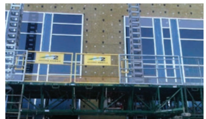
Behind cladding over steel stud walls
