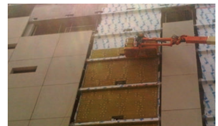
Behind cladding over concrete block walls
