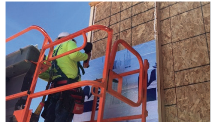
Behind cladding over wood stud walls
