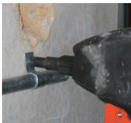
12HSMP034 clip assembly used to secure conduit
