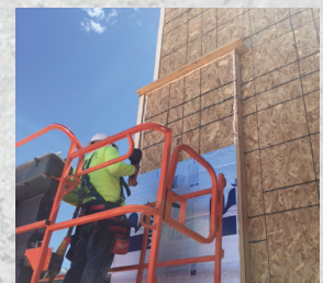
Behind cladding over wood stud walls
