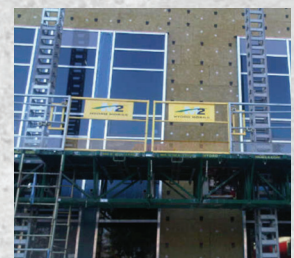
Behind cladding over steel stud walls
