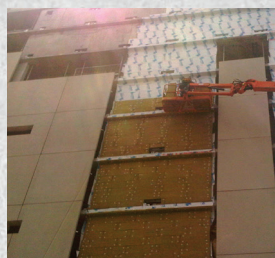
Behind cladding over concrete block walls
