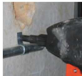
12HSMPO34 clip assembly used to secure conduit
