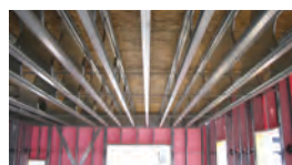
OSB and plywood to I-SPAN joists
