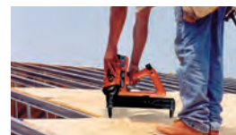
Plywood attachment—using TrakFast plywood to steel pin
