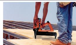
Plywood attachment—using TrakFast plywood to steel pin
