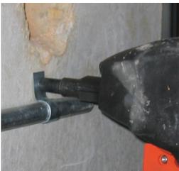
12HSMP034 clip assembly used to secure conduit
