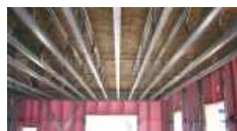
OSB and plywood to iSPAN joists
