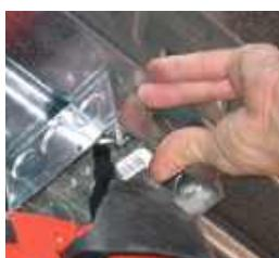
M100 fastener used to attach a junction box
