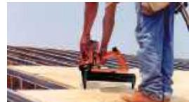
Plywood attachment—using TrakFast plywood to steel pin
