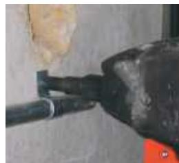
12HSMP034 clip assembly used to secure conduit
