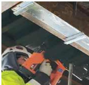
The T4 has enough power to fasten into hard concrete and steel and still will not blow through hollow block.
