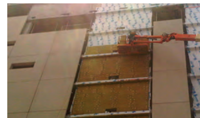
Behind cladding over concrete block walls
