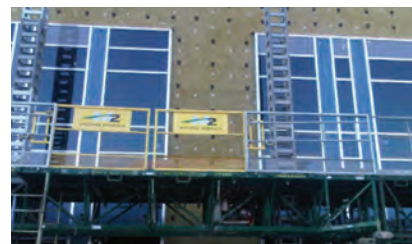
Behind cladding over steel stud walls
