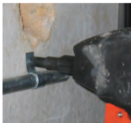
12HSMPO34 clip assembly used to secure conduit
