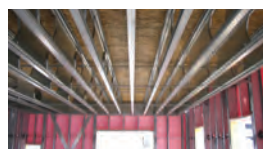
OSB and plywood to I-SPAN joists
