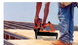
Plywood attachment—using TrakFast plywood to steel pin
